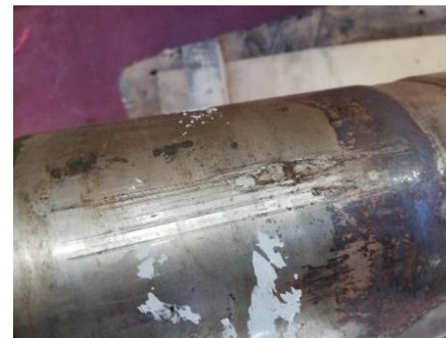
Wear and tear on shaft
